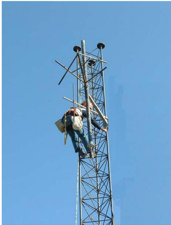
Here a Penetrator is mounted on the full scale tower section mounted to the turntable for testing. This particular order was to optimize the vertical radiation component while leaving the horizontal energy as omni as possible. Notice the vertical only reflectors just over the technician's shoulder. The sample tower section is the exclusive Jampro FMT (Frequency Matched Tower) to minimize tower effects on the station's coverage.
